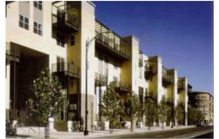
100 Dwelling Units per Acre Downtown San José 5-story stacked townhouses and flats over 2 levels of podium parking.
