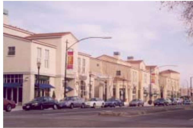
45 Dwelling Units per Acre Avalon, San José 3-story stacked units over retail with podium parking.
