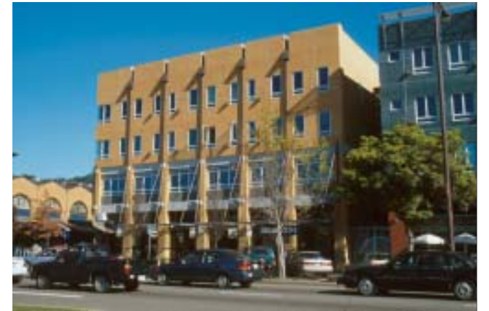
Mixed-Use Building Shattuck Ave., Berkeley Apartments over offices over retail.
