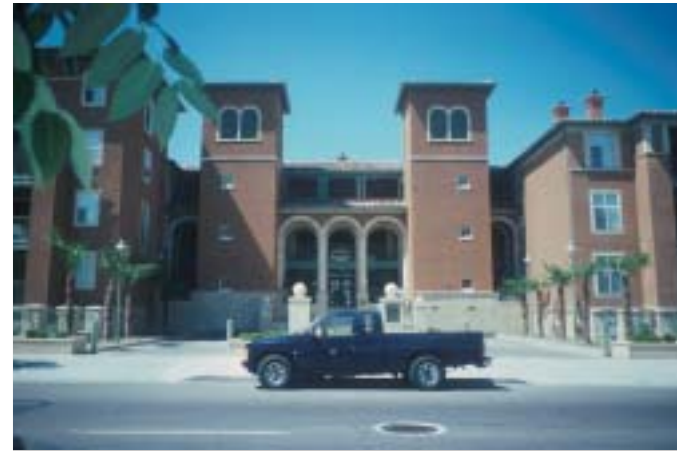
75 Dwelling Units per Acre Villa Torino, San José 4-story stacked flats over two levels of podium parking.
