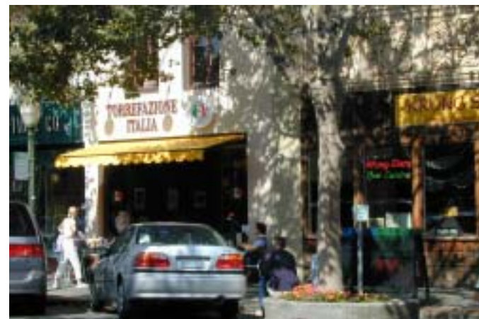
Offices over Retail University Ave, Palo Alto Offices over retail, structured parking.
