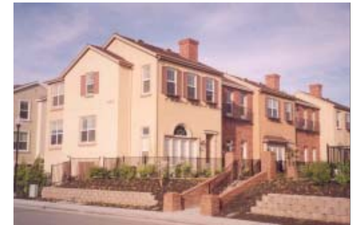
27 Dwelling Units per Acre Georgetown, San José “Tuck Under” townhouses with alley access to garages at the rear
